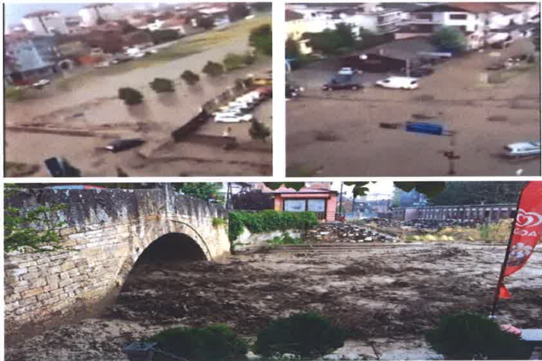
Fig. 2. Flooding in Tetovo on 3 August 2016 and flood damage along the Pena River
